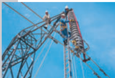
Utilities and process control centers
